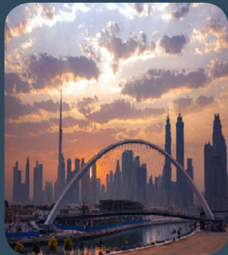
Dubai Water Canal
